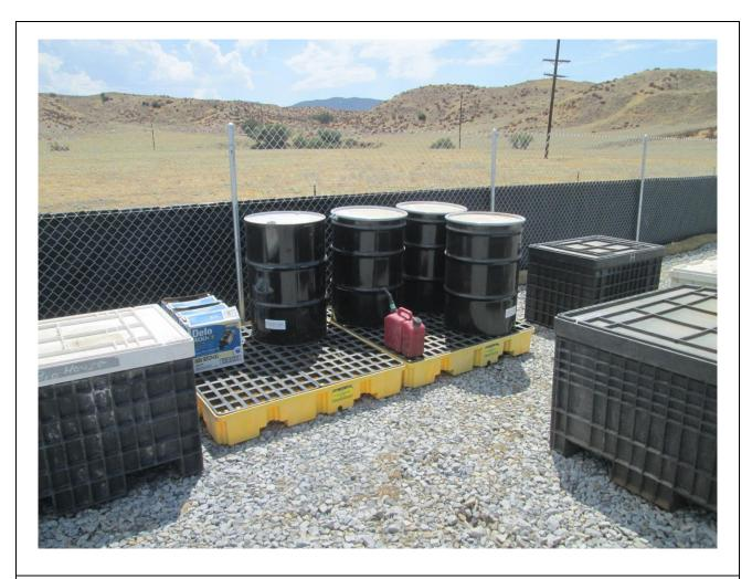
**Photo 5:** At Warner Substation Staging Yard (TL 682), hazardous materials were observed being stored above catchment pallets in accordance with the SWPPP and MM PHS-2.
