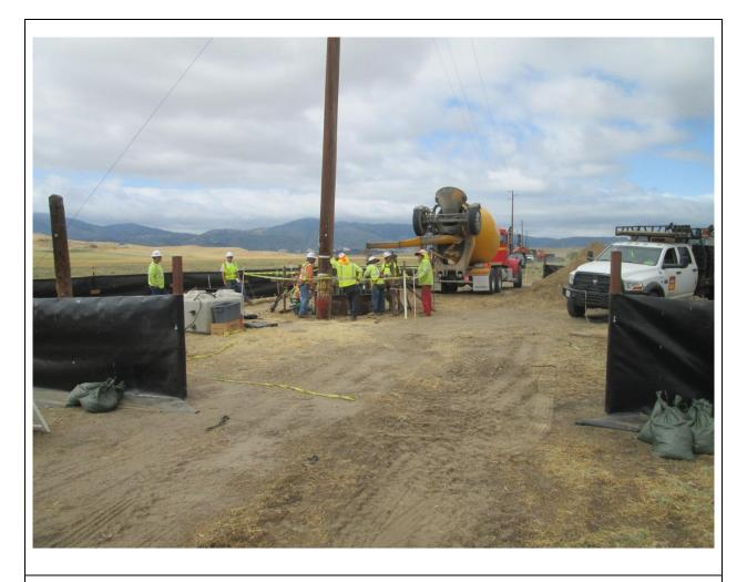
**Photo 2:** A construction crew observed pouring concrete during conventional foundation construction at Pole Z118232 (TL 682). Stephens' kangaroo rat exclusion barrier was observed around the perimeter of the workspace in accordance with MM BIO-31.
