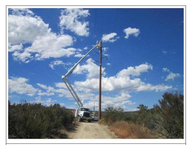
**Photo 1**: A construction crew observed conducting overhead line work in preparation for wire stringing activities at Pole Z44247 (TL 6931).
