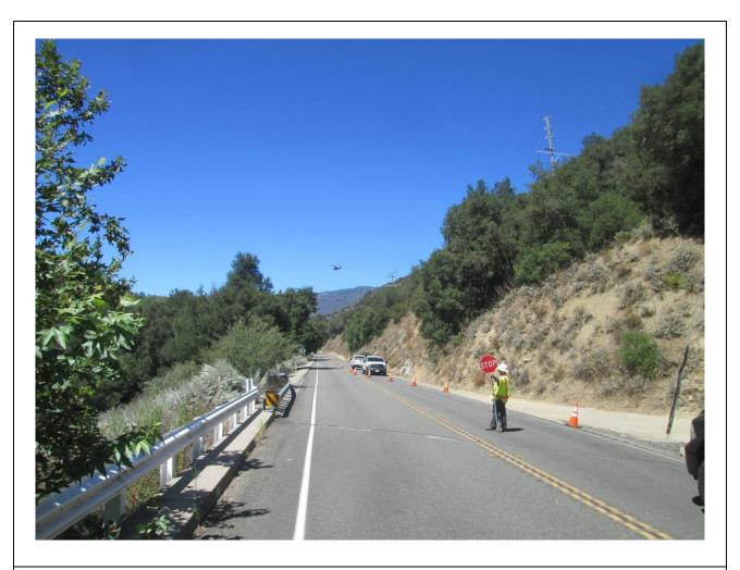
**Photo 6:** During helicopter external load operations assisting in transport of materials and equipment used in foundation drilling and grouting along TL 682, traffic control notification signs, cones, and flagpersons were utilized to temporarily stop traffic when loads were transported over Highway 76 (APM TRANS-02).
